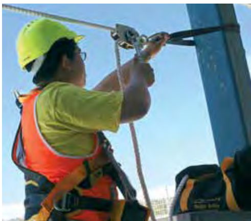
Rope temporary life line being installed and tensioned.
