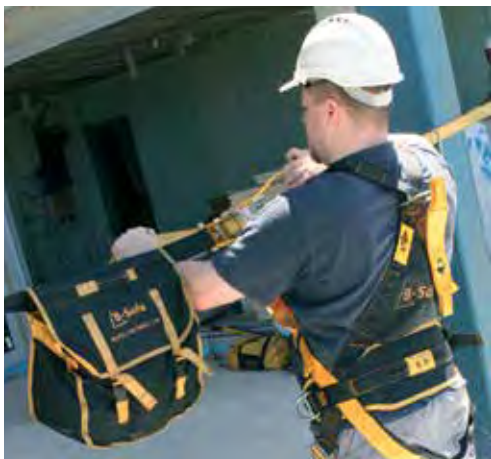
Web temporary life line, ratchet tensioning method.
